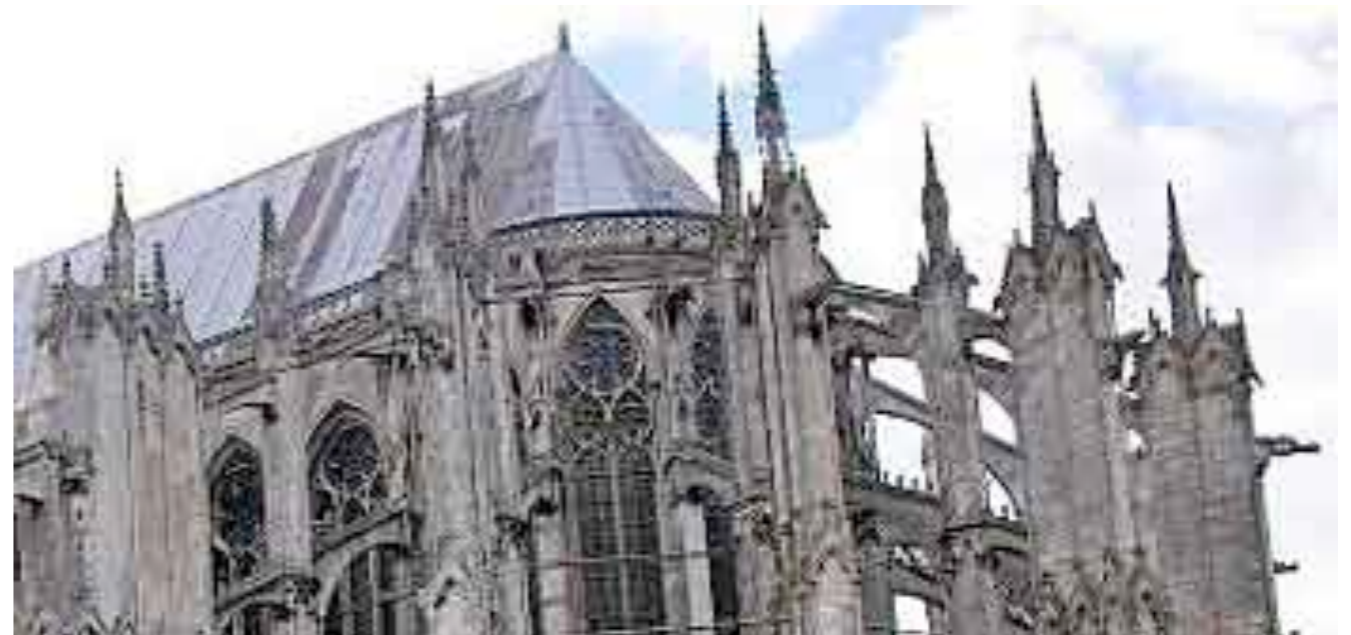
Beauvais Cathedral (~300 years to build, at least 2 collapses)
